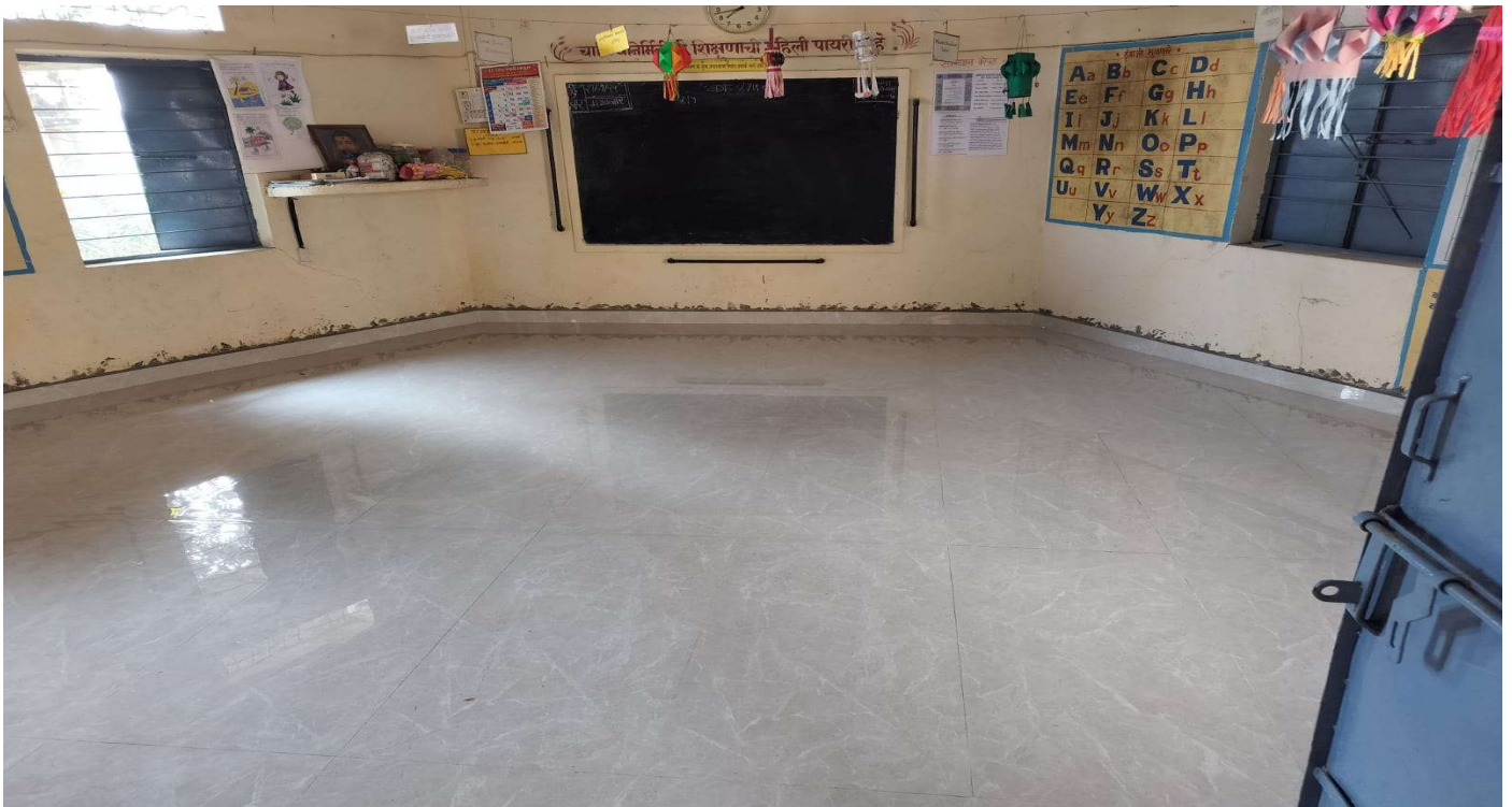
Classroom Flooring construction at the Zilla Parishad School.
